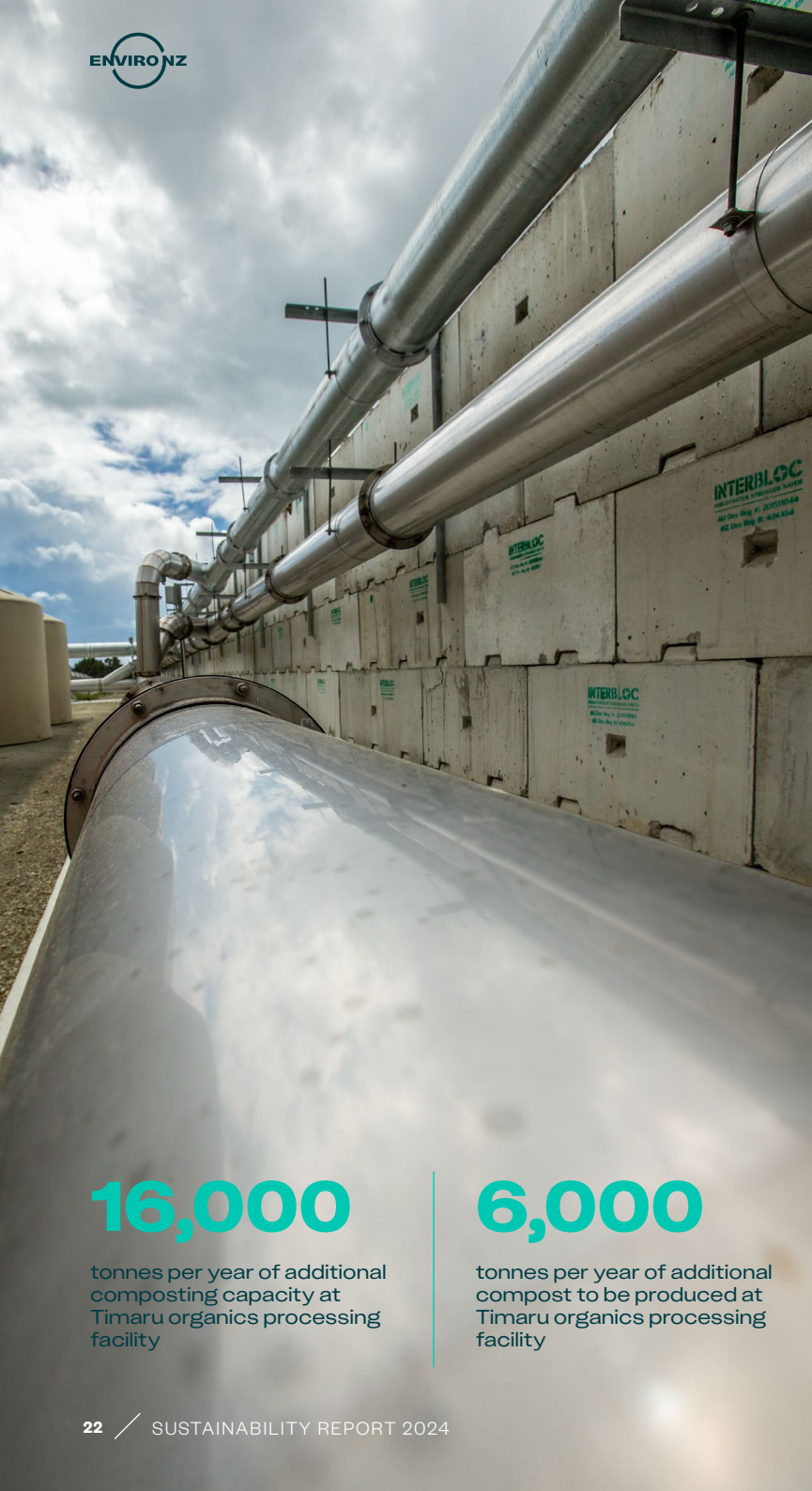
LEFT Aeration pipes at Timaru organics processing facility.
