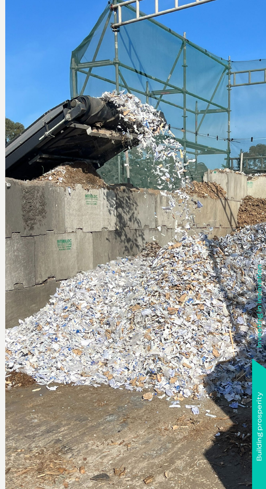
RIGHT Plastic shredding at Golden Bay Cement.
